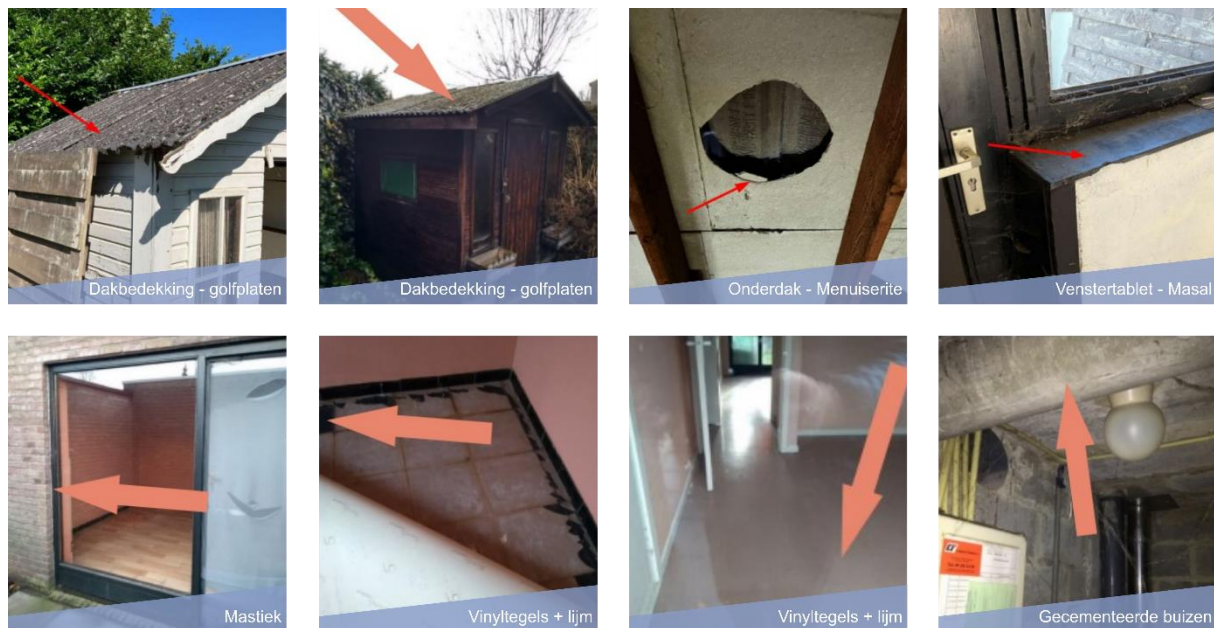
Figuur 38: Asbestoepassingen patrimonium SHM's (Boydens, 03/01/2020; Pede, 23/06/2022)
