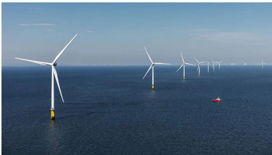
Figure 10 Hornsea 2 wind farm in the UK, with 1.3 GW capacity. Ref.: [83]
