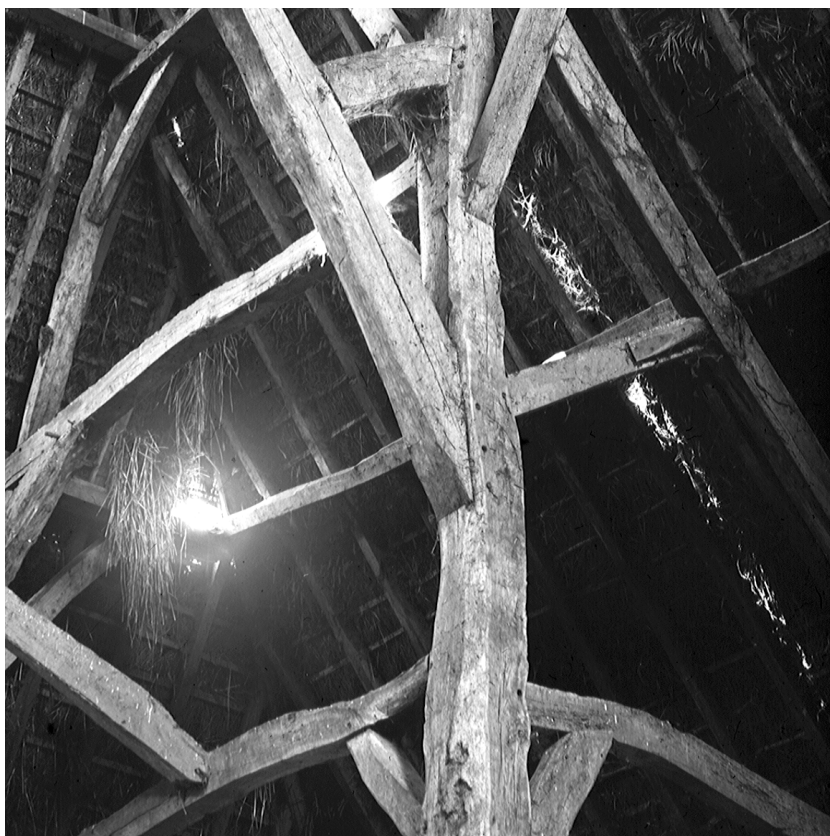
Fig.8: Pen-en-gat verbinding
