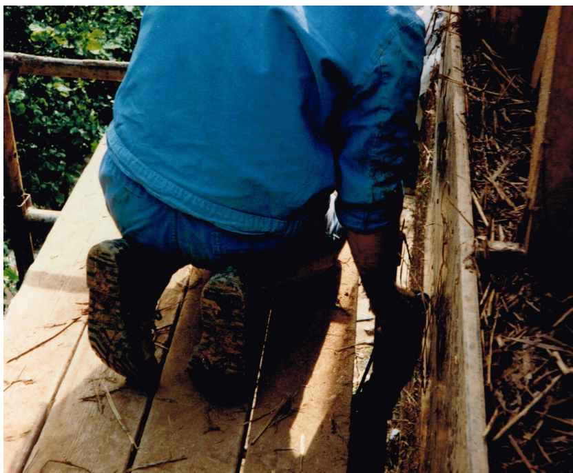
Fig.57: Wand C: schuifbekisting
