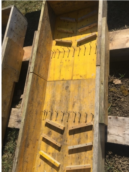
Figure 3. Boxes ready with the screws and wood
