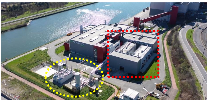
Figure 2. 1. Aerial view of the anaerobic digestion plant in Uvélia. The two digesters are outlined by the red square and the cogeneration engines are circled in yellow. Source: Image captured from a video created by the company Greg Bugni créateur d'images.
