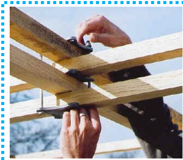
Figuur 3-42: Stalen klemverbinding [17]
