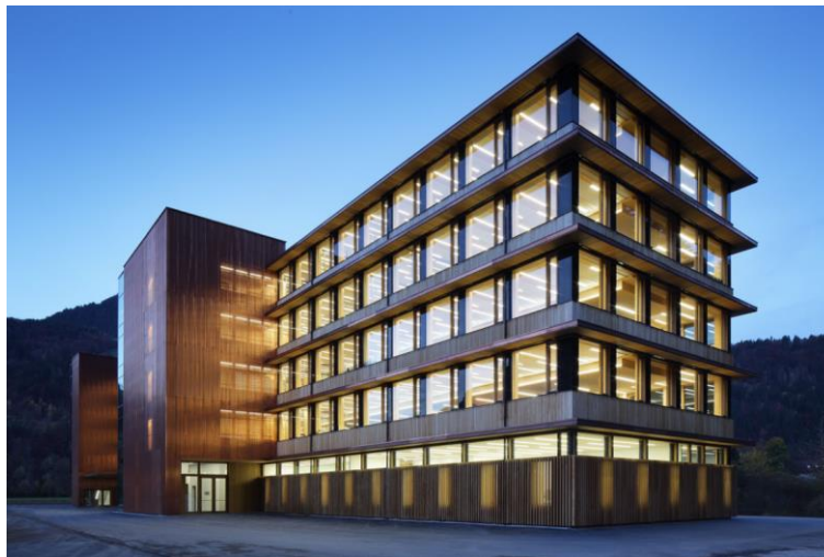
Figure 3: Hybrid concrete-timber structure: Illwerke Zentrum Montafon, Austria [11]
