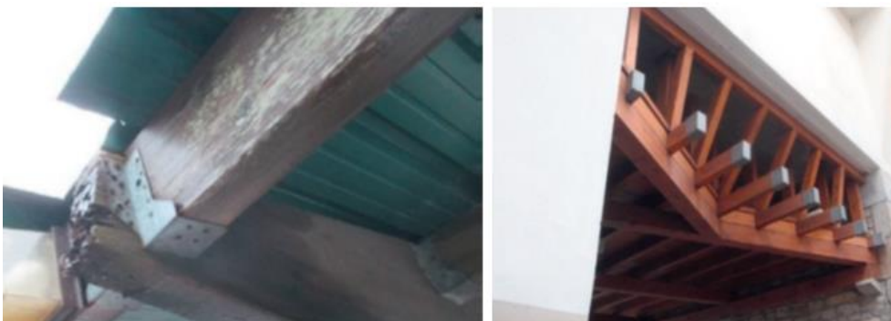
Figure 16: Design rule 3: provide an end grain protection
