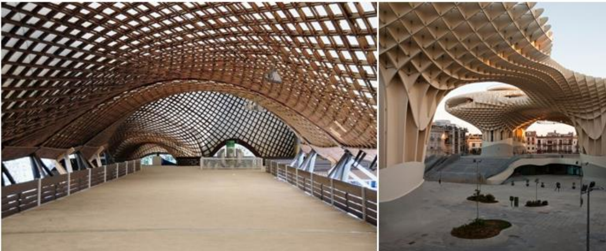
Figure 4: Mannheim Multihalle, wooden roof structure (left); Metropol Parasol, Seville (right) [12], [13]
