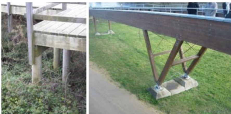
Figure 19: Design rule 6: avoid direct ground contact
