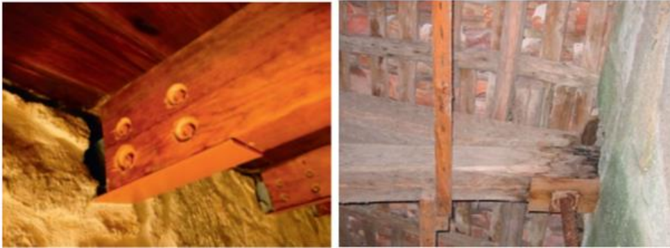
Figure 14: Design rule 1: avoid direct contact with wet walls [10]
