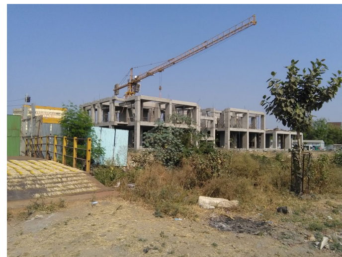
Figure 69. Image of Chikhali building site
