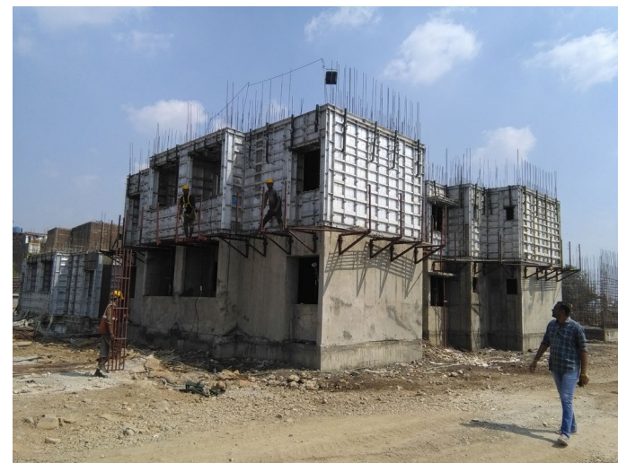
Figure 67. Image of Wanjari building site
