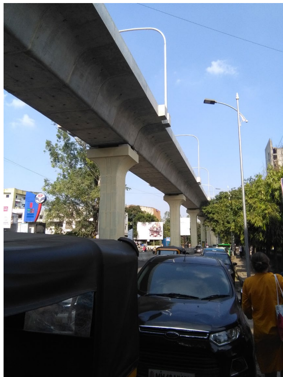
Figure 12. Picture of Nagpur Metro rail
