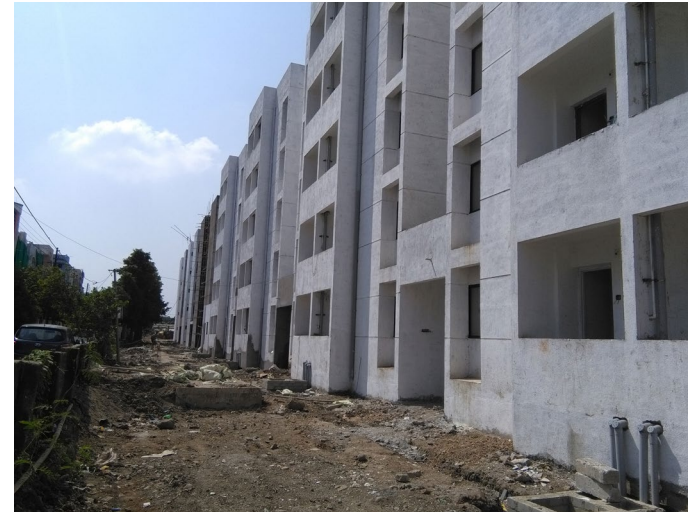
Figure 65. Image of Wathoda building site
