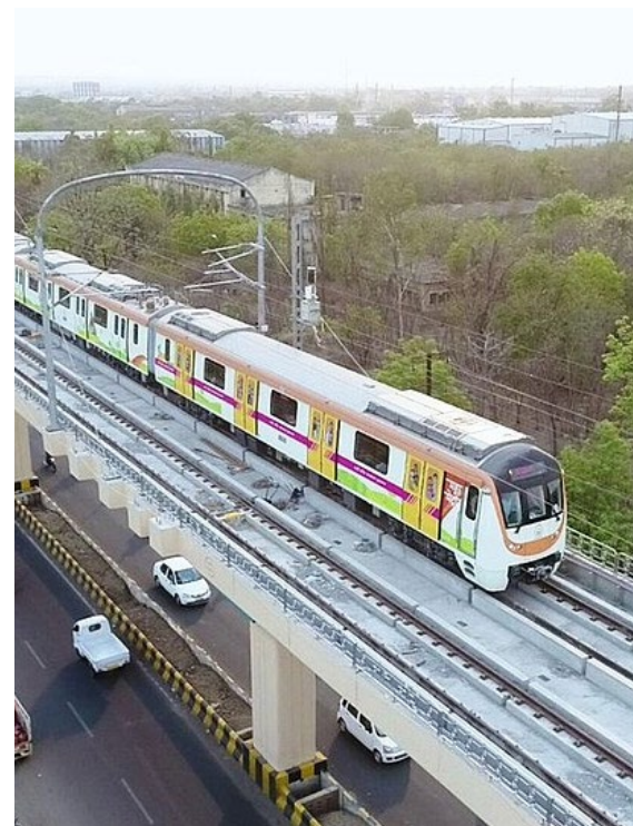
Figure 13. Picture of Nagpur Metro Image of www.metrotrainnagpur.com
