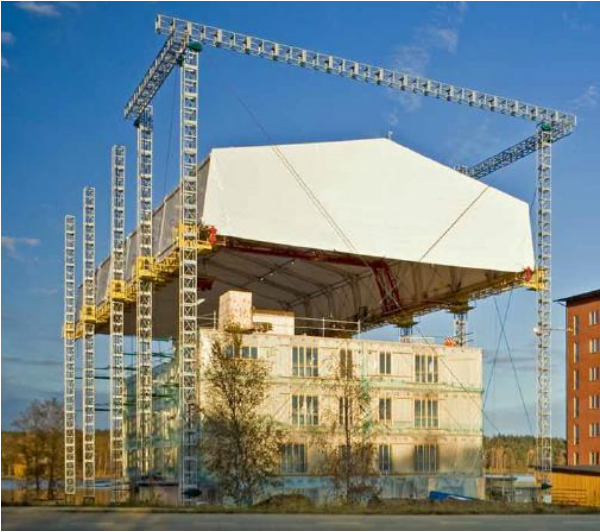
Figure 7 – Temporary protective roofing at a construction site [4]
