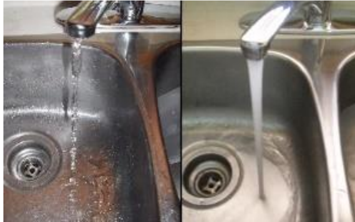
Fig. 3.10: Comparison between water flow without and with aerator Source: www.eureka4you.com
