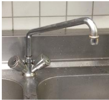
Fig. 2.12: Double handle faucet located in the kitchen
