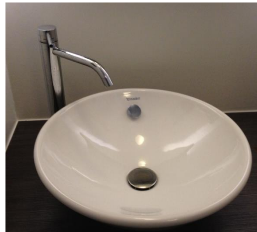
Fig. 2.20: Sink located in public restroom
