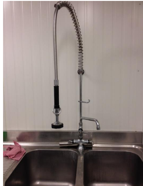
Fig. 2.3: Pre-rinse spray used in Bossuwè
