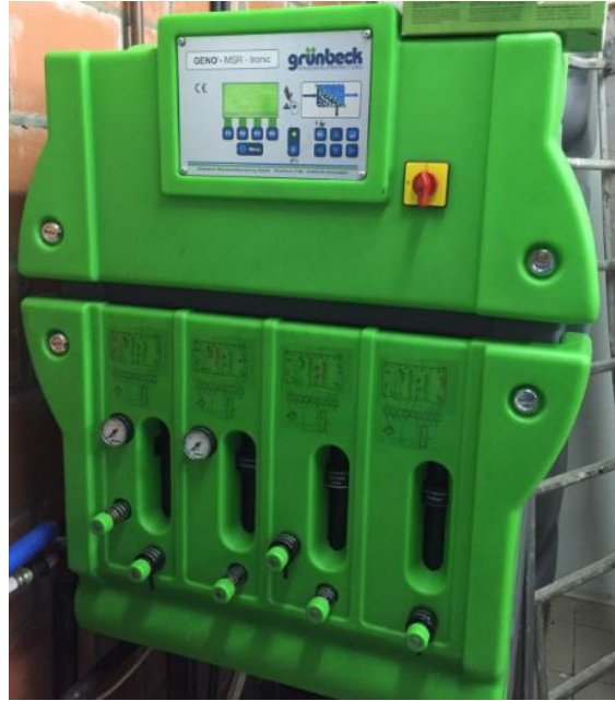
Fig. 2.18: Iron remover
