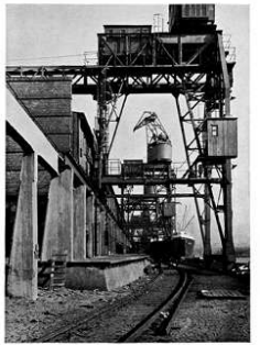
Large industrial structure with steel beams Large industrial structure with steel beams
