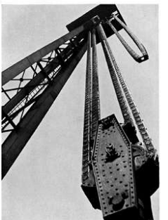
Large industrial structure with steel beams Large industrial structure with steel beams
