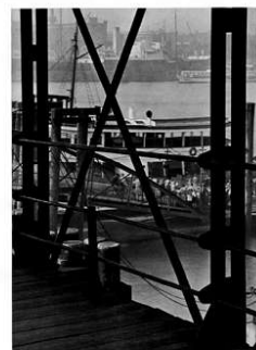
Steel beams on the deck Steel beams on the deck
