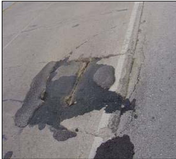
Figuur 20: Punch-out in DGB [25]
