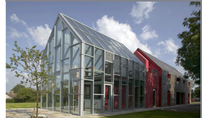
Figuur 2.10_Sliding House < dRMM-Architecture ( www.drmm.co.uk+dRMM/news.html )
