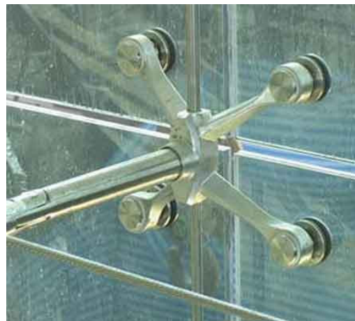
Figuur 25: 4-puntsbevestiging van Spider Glass (© www.anzor.co.nz )
