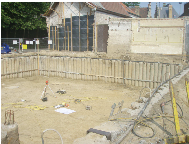
Picture 1: Pile wall
