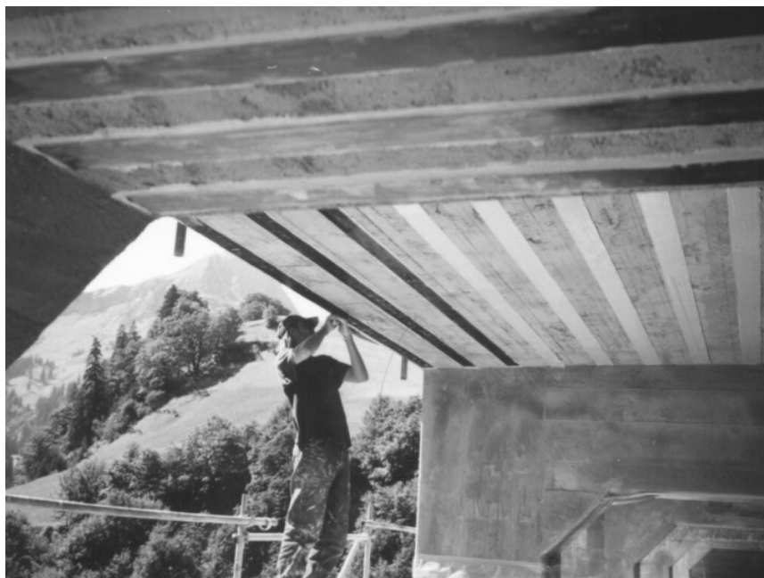
Fig. 1-7 Strengthening with FRP EBR of the Tannberg bridge in Austria
