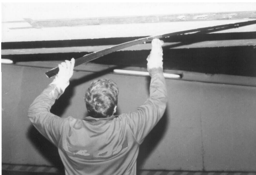
Fig. 2-6 Application of a prefabricated FRP EBR system
