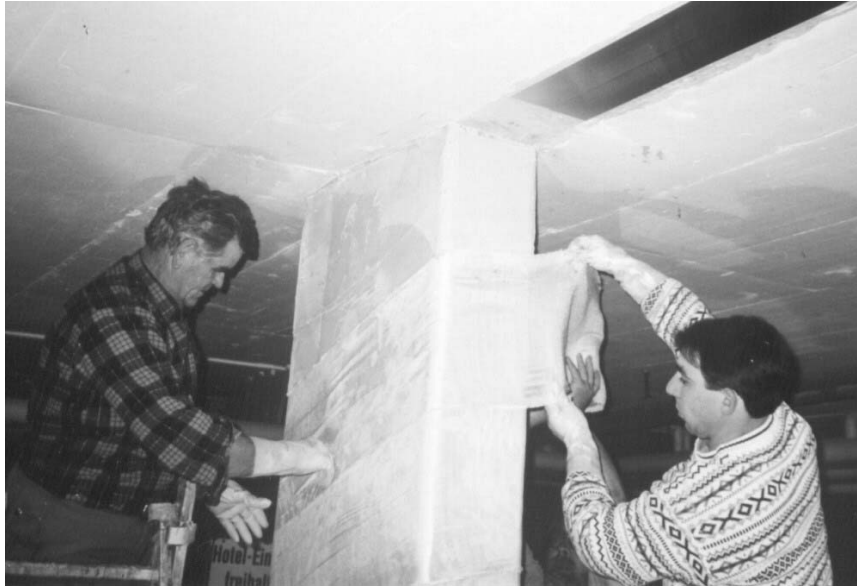
Fig. 2-7 Application of a wet lay-up FRP EBR system
