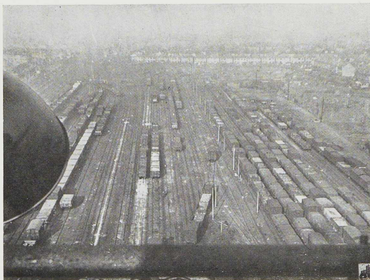
(Photos Southern Railway.)
